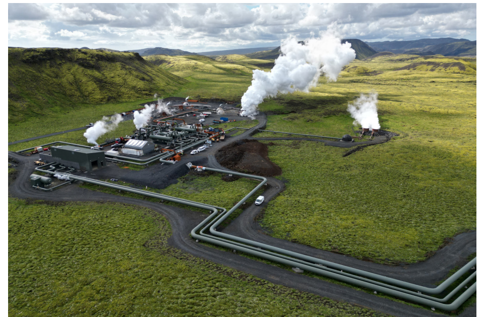
Washing tower for Carbfix, 2022
